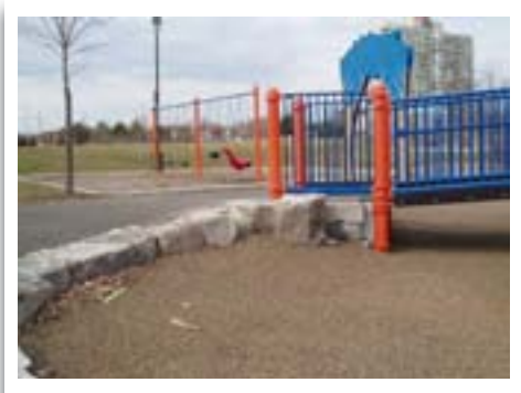
Using grading to provide access to raised play area. PHOTO COURTESY OF SHIRA STANDFIELD
