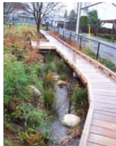
Raingarden with boardwalk for circulation and discovery. PHOTO COURTESY OF STEFUIK
